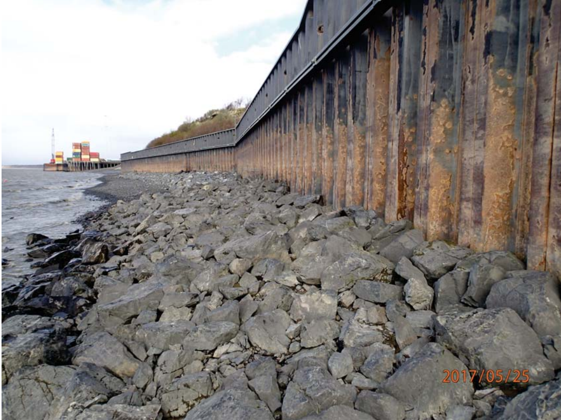
STA 21+00, Riprap @ Toe, Facing Downstream, May 2017
