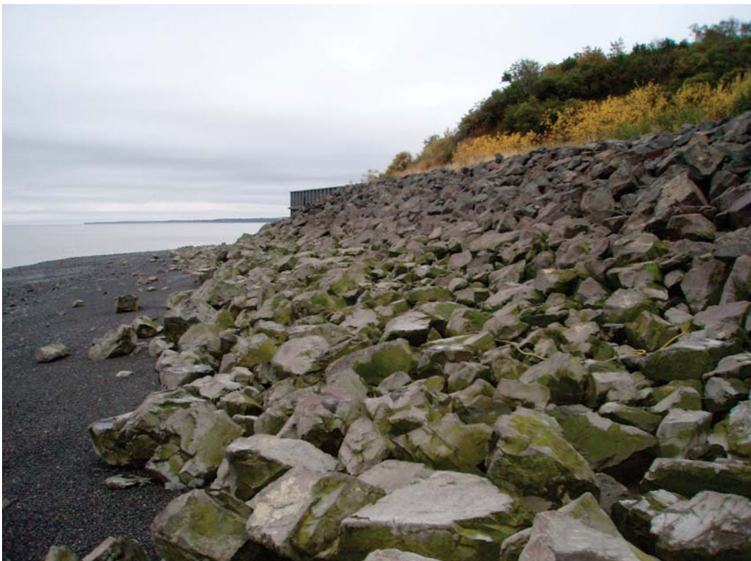
Rip-rap protection at the eastern extent of bank stabilization, 14 August 2008
