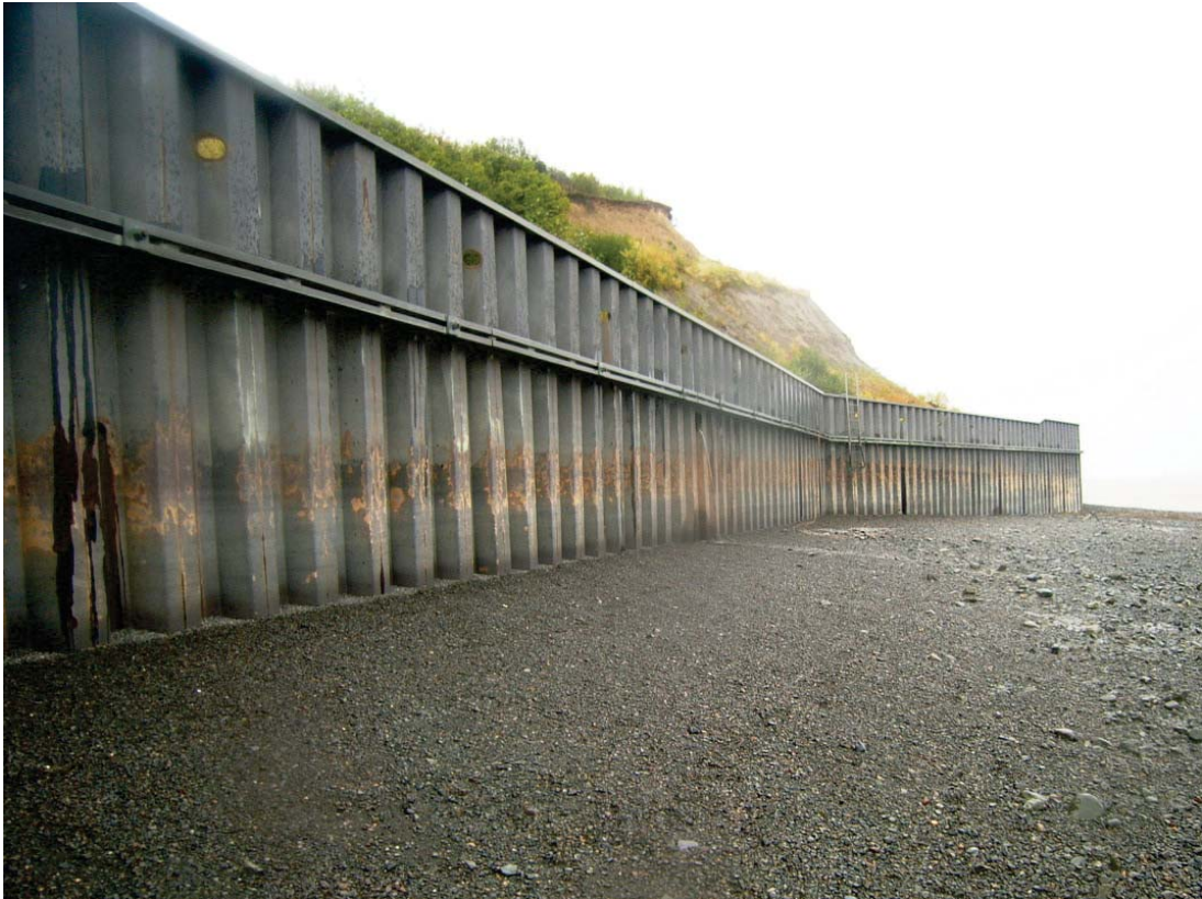
H-pile supported sheetpile bulkhead, September 2008
