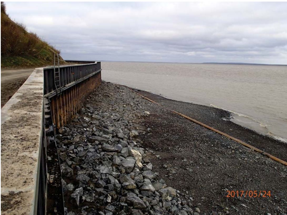
Top of Wall, STA 19+10, Riprap @ Toe, Facing Upstream, May 2017
