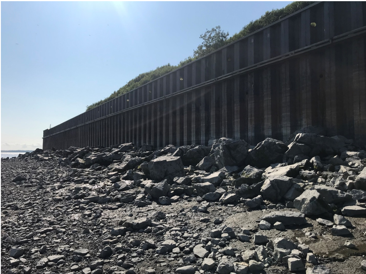
Figure 4. Sheet Pile Wall on Dillingham Waterfront.
