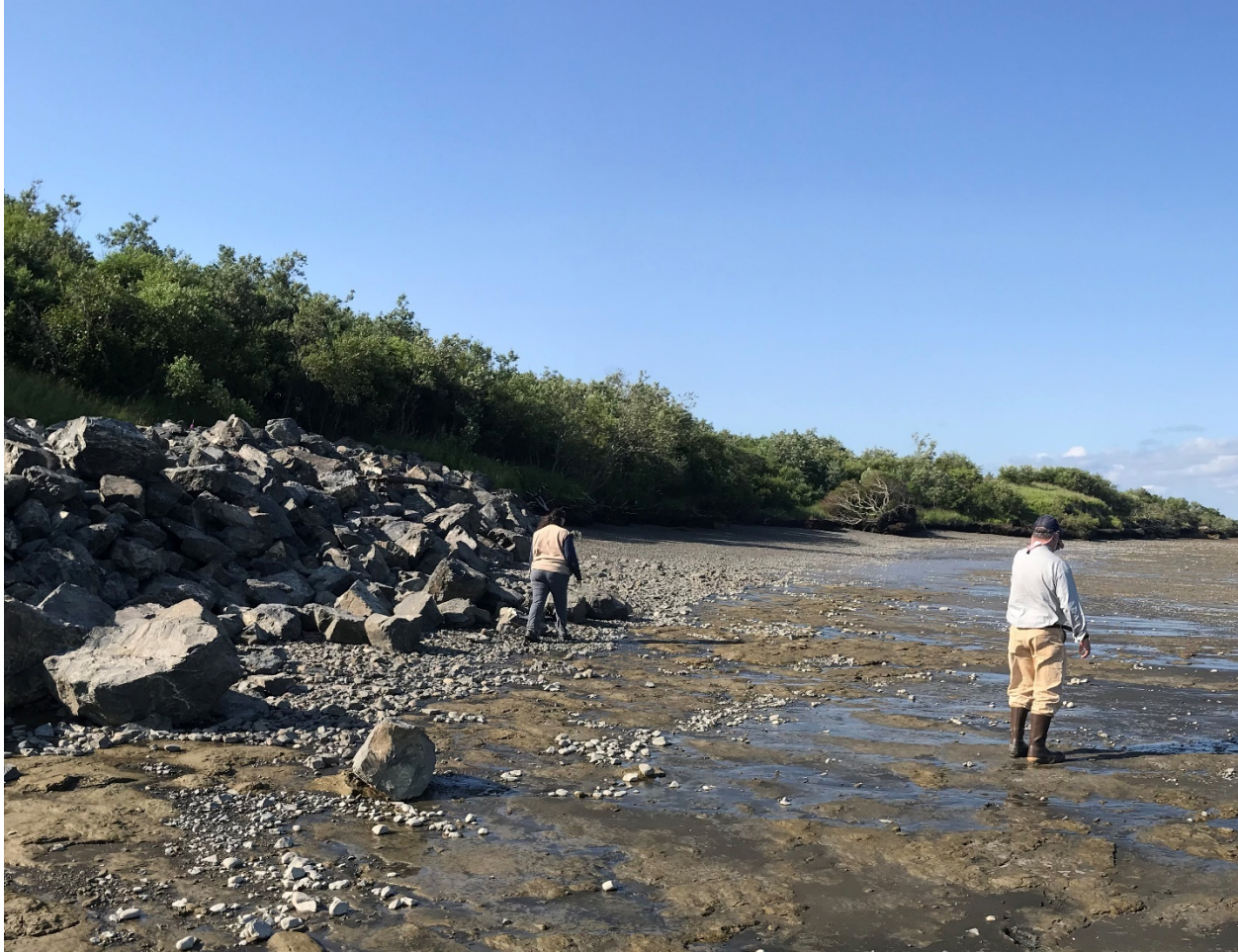
Figure 3. Rock Revetment Adjacent to the Project Site.
