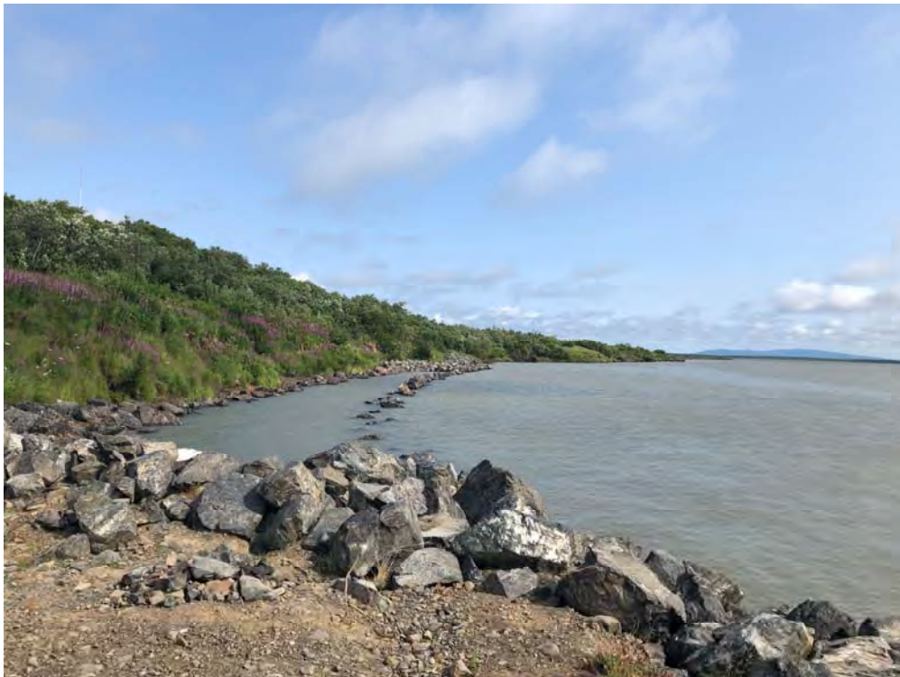
Photo 2 – Bank Armoring/Access Road (Looking North from Outfall at High Tide)
