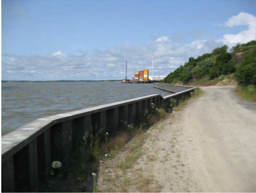
Photo 3 – Sheetpile Wall (Looking Southwest from Outfall at High Tide)
