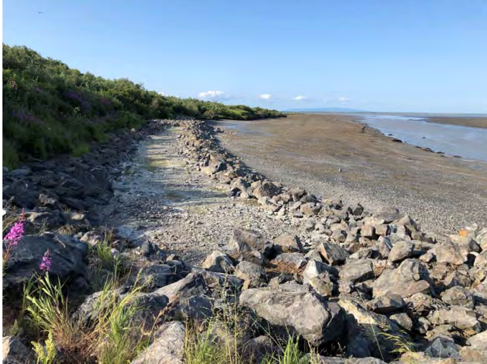
Photo 11 - Bank Armoring/Access Road (Looking North from Outfall at Low Tide)
