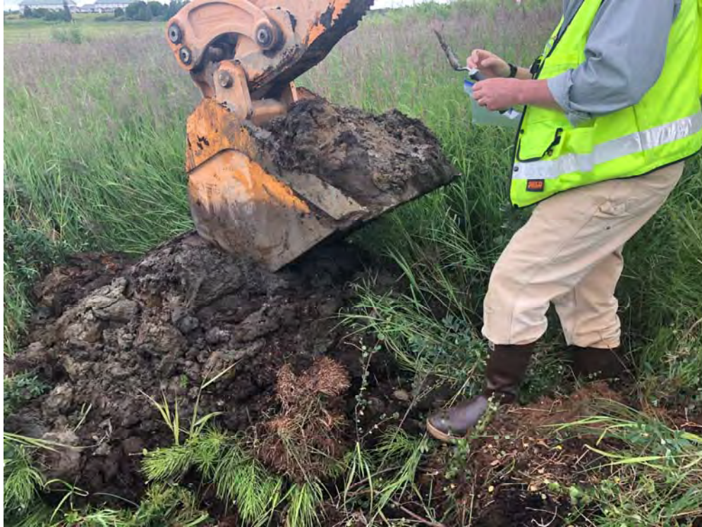
Photo 15 - Site 2 Test Pit (Northwest Side of City Shop Pad)
