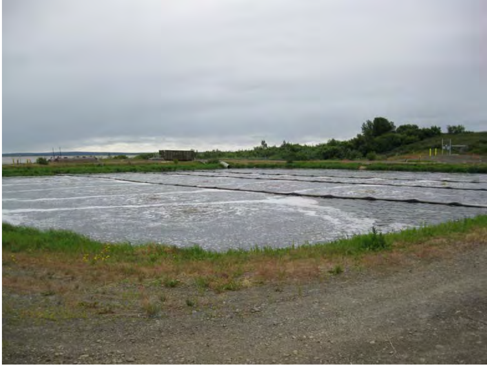
Photo 13 - Cell #1 Aeration (Looking Southeast)
