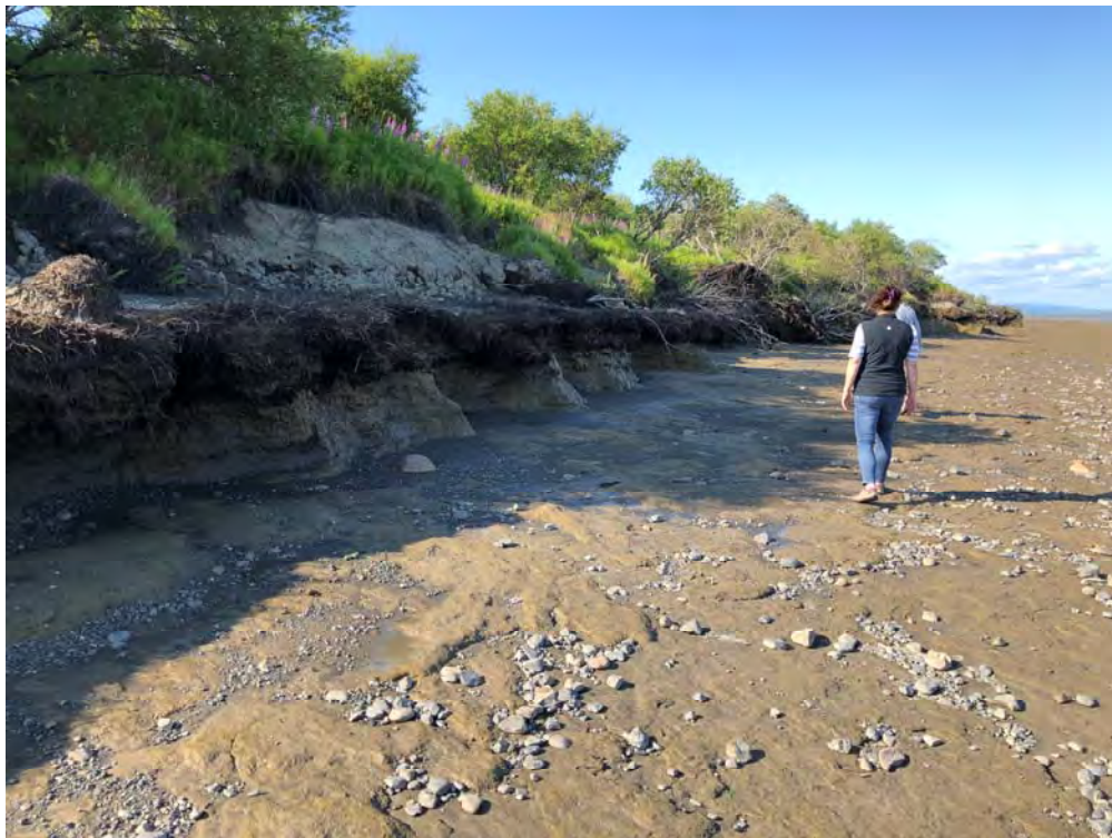
Photo 12 – Bank/Bluff (Looking North Adjacent to Lagoon)
