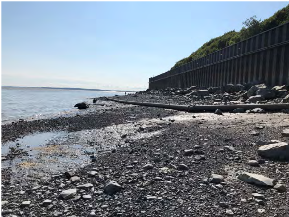
Photo 8 - Sheetpile Wall (Looking Southwest from Outfall at Low Tide)
