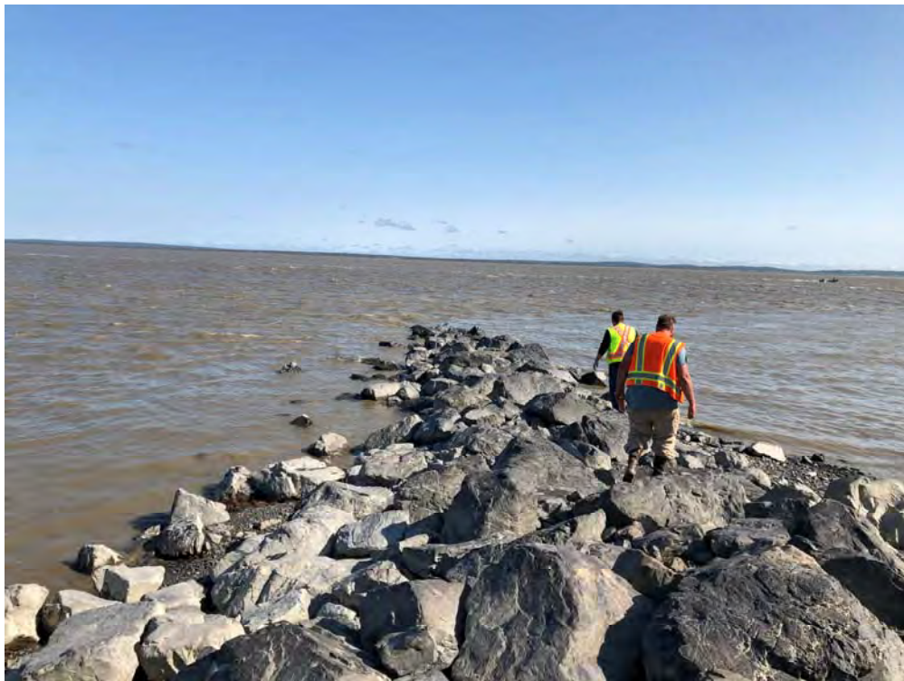
Photo 10 - Foremain Outfall Armoring (Looking East at Low Tide)
