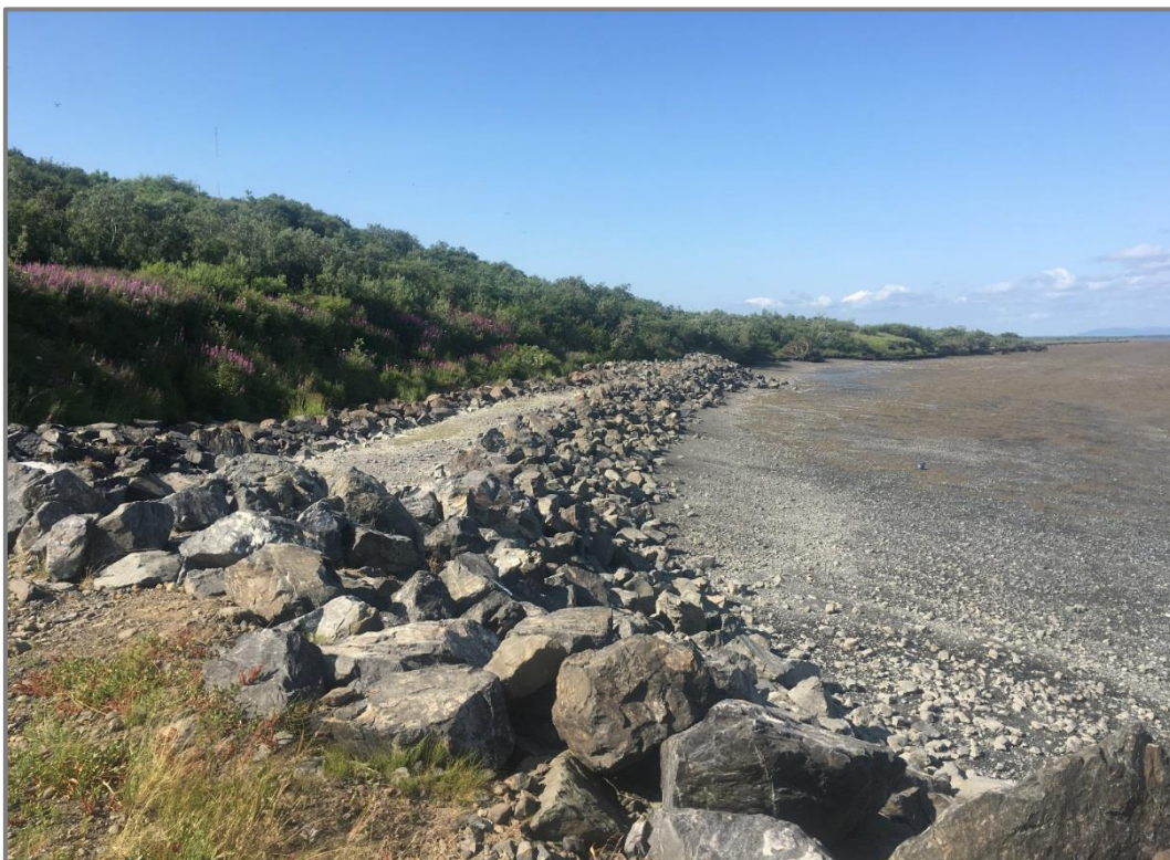
Existing Lagoon Site, General Beachline Conditions and Locally Available Armor Rock, View NE
