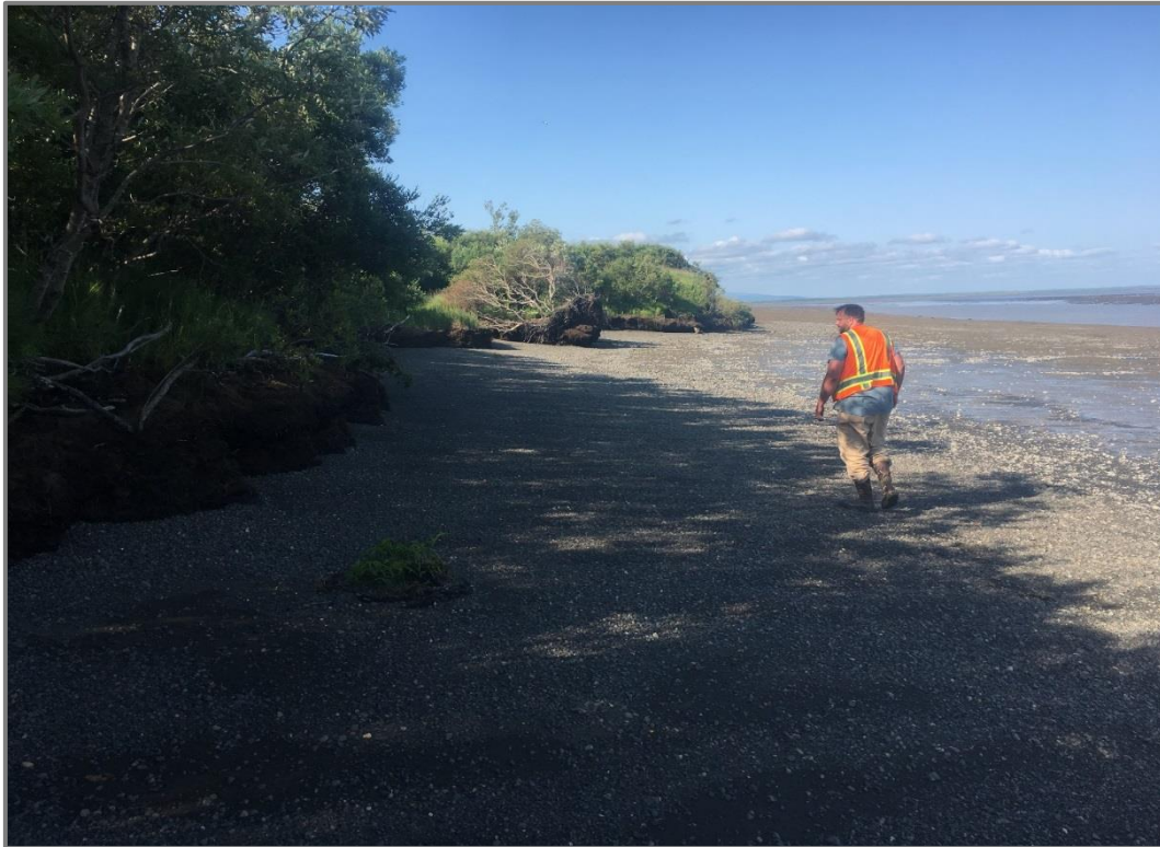
Existing Lagoon Site, Beachline Conditions Showing Organic Mat Along Unarmoured Facing, View NE
