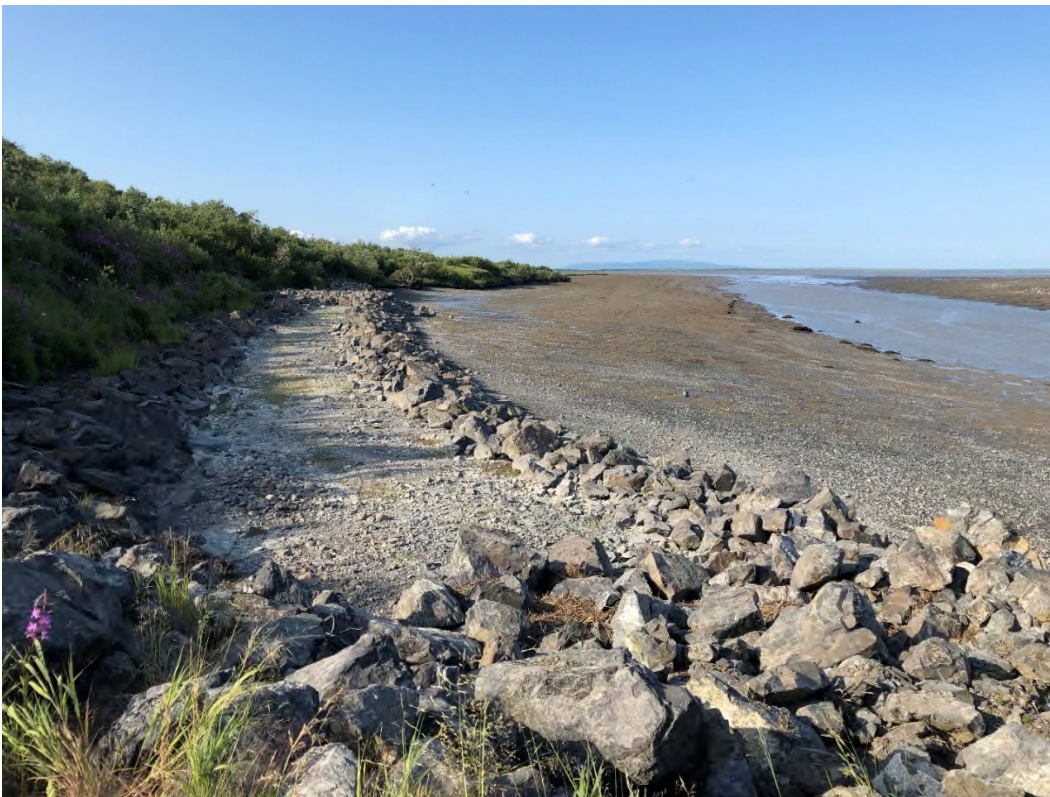
PHOTOGRAPH 2 – EFFLUENT LINE PROTECTION NORTH OF OUTFALL (7/11/19)
