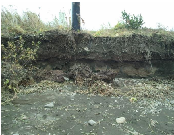
East side of Dillingham harbor after 2009 storm
