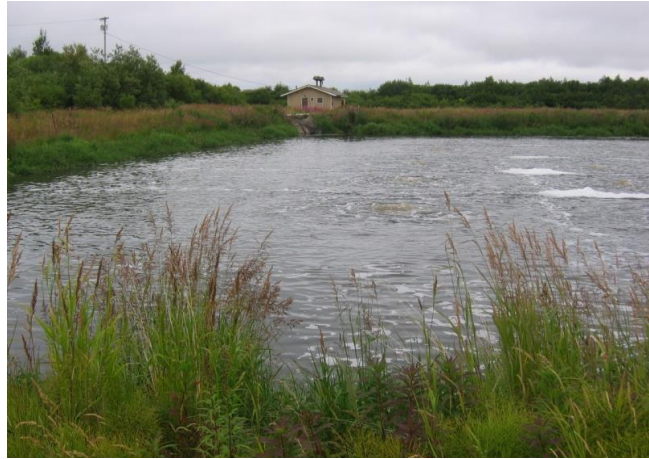
Figure 1 Wastewater Treatment Lagoon
