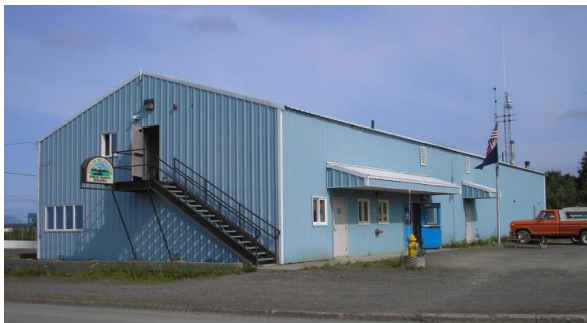
Figure 3 Public Safety Building
