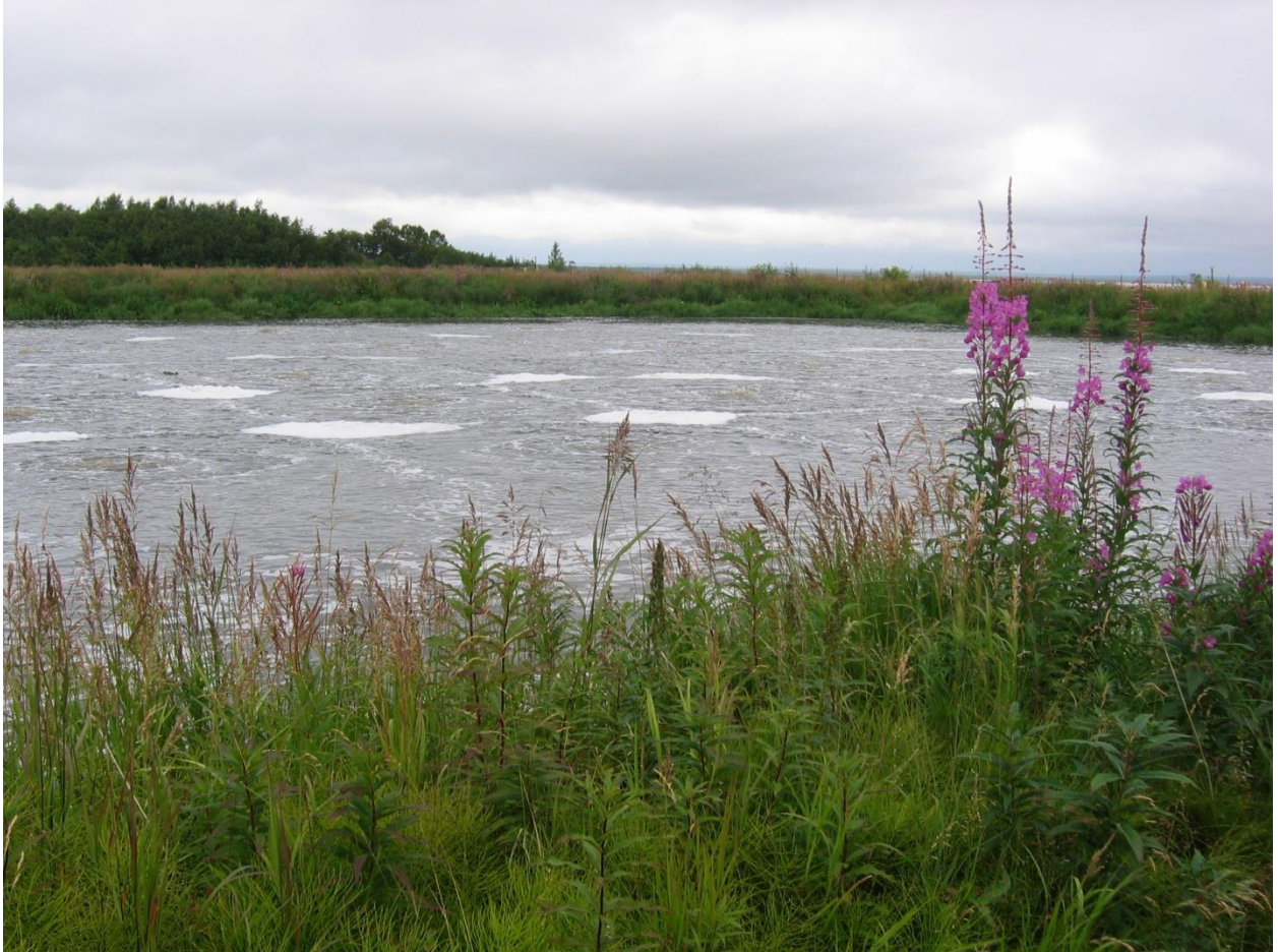
Dillingham wastewater treatment lagoon.
