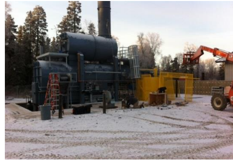
Figure 2 Dillingham Landfill Incinerator
