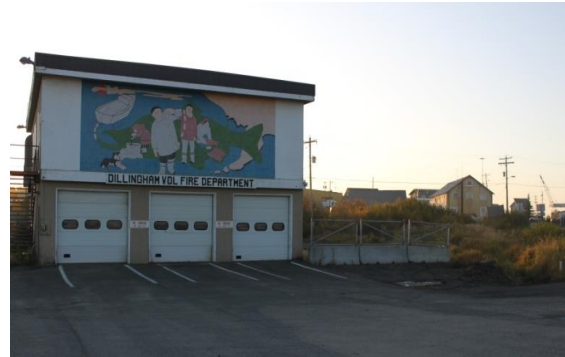
Downtown Fire Hall bays are too small for new equipment.
