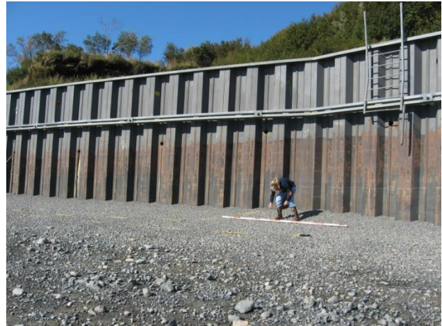
Snag Point Bulkhead
