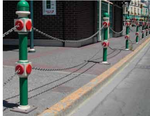
Figure 8. Example of Decorative Bollard and Chain Fencing in Victoria, BC. (Photo by Norm Ringuette, 2007).
