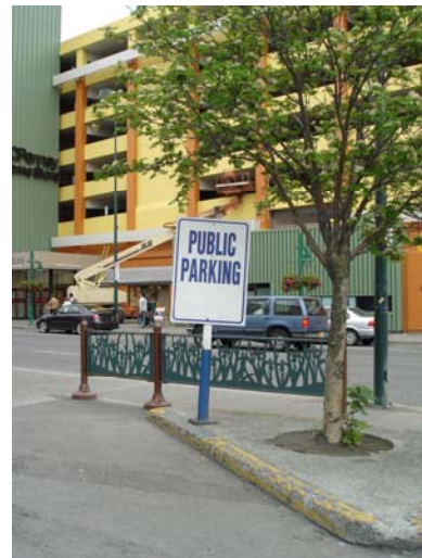
Figure 9. Example of a decorative fence used to separate a sidewalk from the adjacent parking area.
