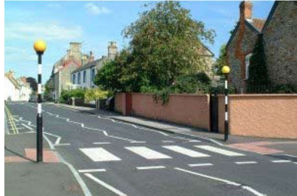
Figure 14. Zebra Crossing with Belisha beacons
