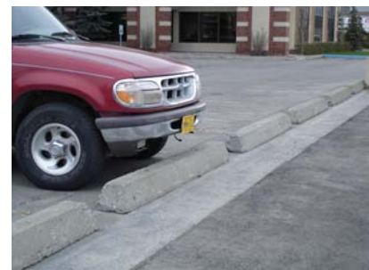
Figure 7. Curb stops used in a parking lot.
