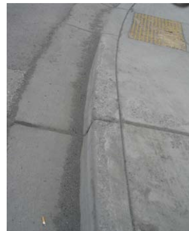
Figure 6. Example of Vertical Curb
